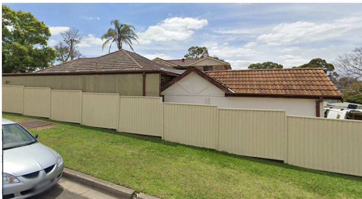
Plate 35: View to the east showing the western boundary of No. 45 Neville Street.
