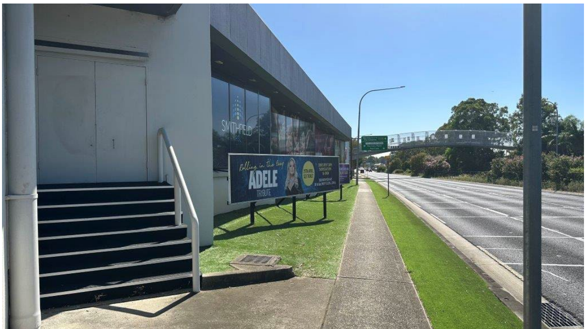
Plate 7: View towards the north-east along the Smithfield Road, frontage.
