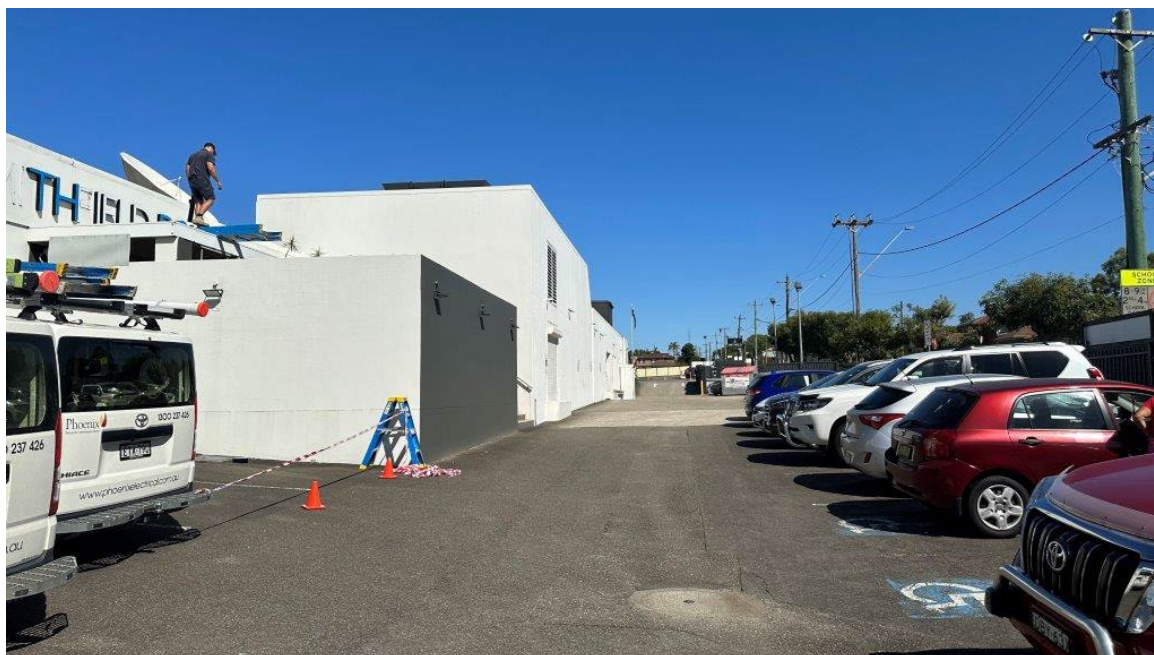
Plate 4: View towards the west along the northern side of the RSL Club Building. Driveway and loading dock.
