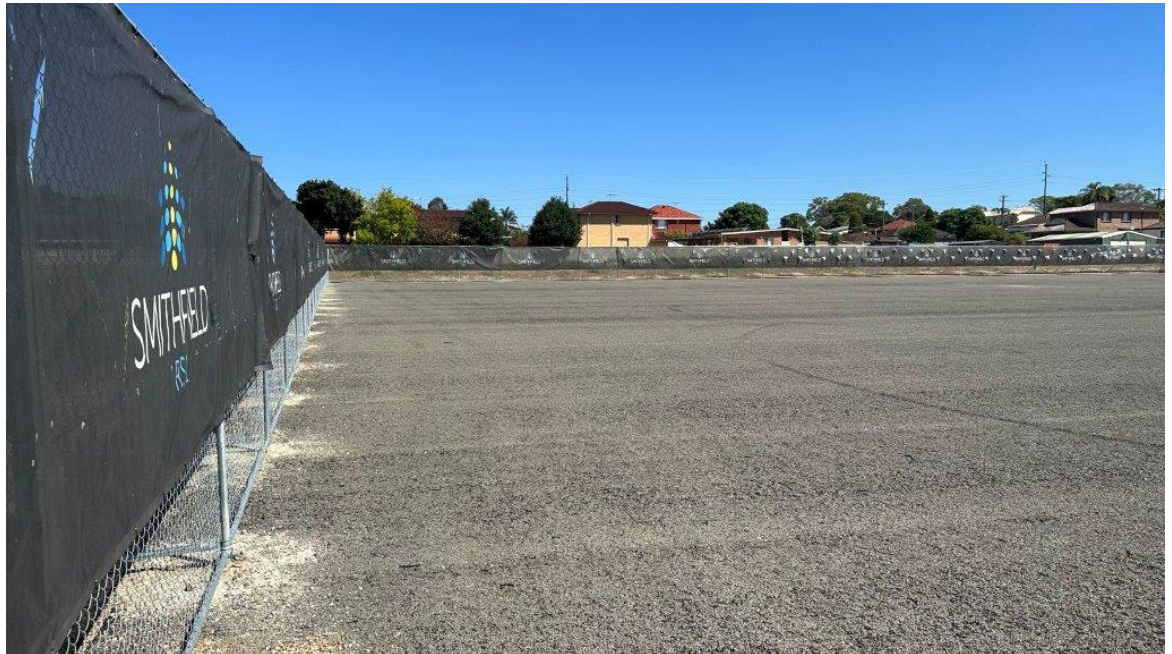
Plate 45: View towards the west across the rear of No. 148, 150a and 152a Brennan Street, showing the recently completed carpark.
