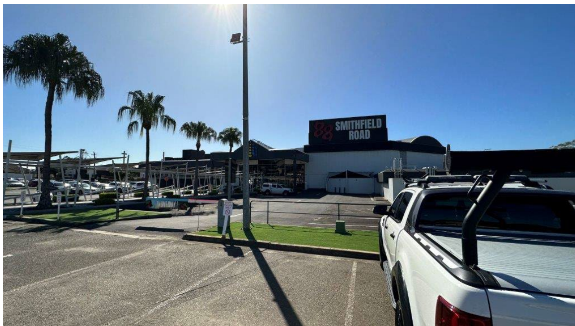
Plate 2: View towards the east from the carpark towards the RSL Club building.
