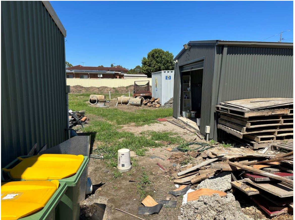
Plate 28: View towards the south across the rear half of No. 41 Neville Street showing scattered waste debris and one of the detached metals sheds and part of the shipping container.
